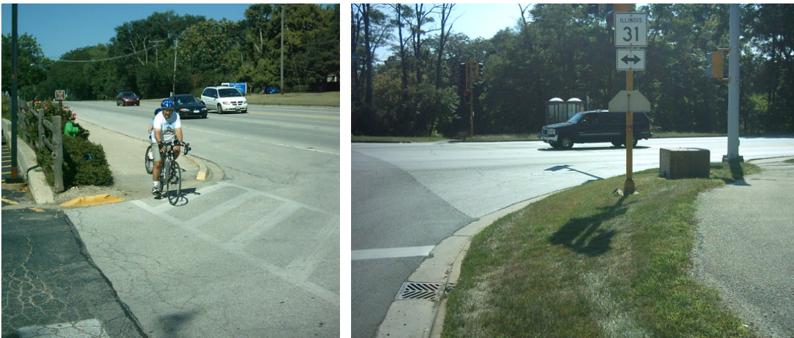
Figure 5.10. Left: Fabyan sidepath at Holmstad entrance. Right: Sidepath at Illinois 31 crossing.
