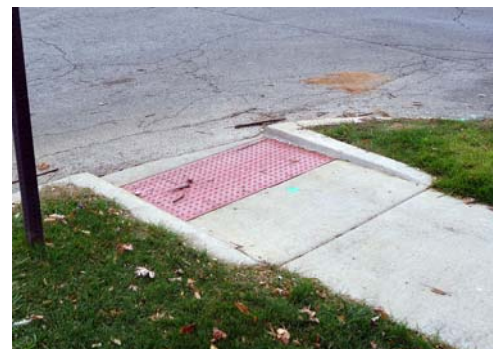
Fully accessible detectable ramp
