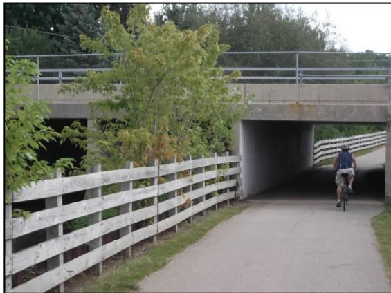
Figure 4.8. Trail underpass of Hershey Road.
