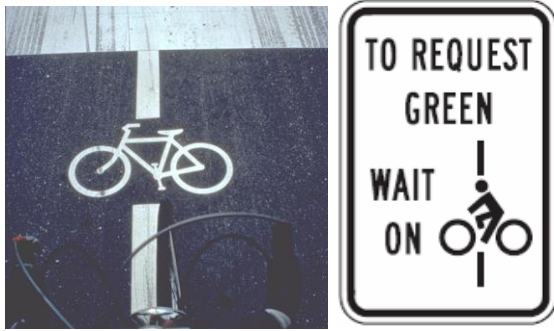
Figure 2.11. Signal activation marking and sign.
