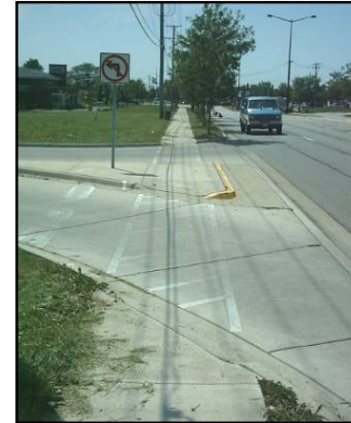
Figure 2 – Left: poor crossing and stop bar placement. Right: good use of a right-in-right-out island
