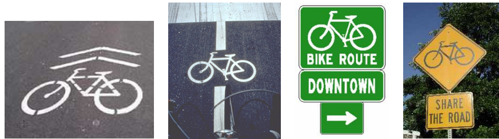
Figure 3 – Pavement Markings and Signage: “Sharrows” – indicates proper bike position in the presence of on-road parking; on-road traffic signal actuation for bicycles; Bike Route signage with wayfinding; Share the Road signage.
