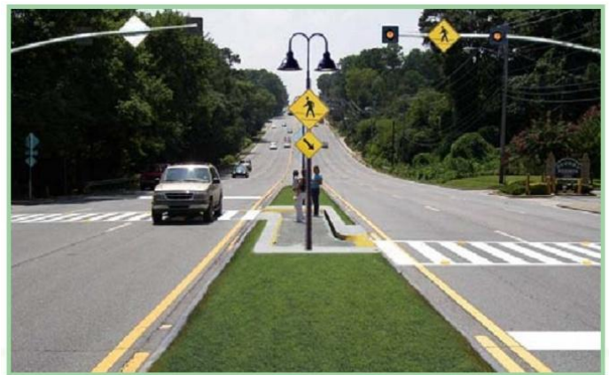
Figure 6 Pedestrian refuge islands break the street crossing into more manageable sections while providing a physical buffer from fast moving traffic. The stop bar is pulled back to help motorists in the inside travel lanes see crosswalk activity. Images courtesy of PBIC.
