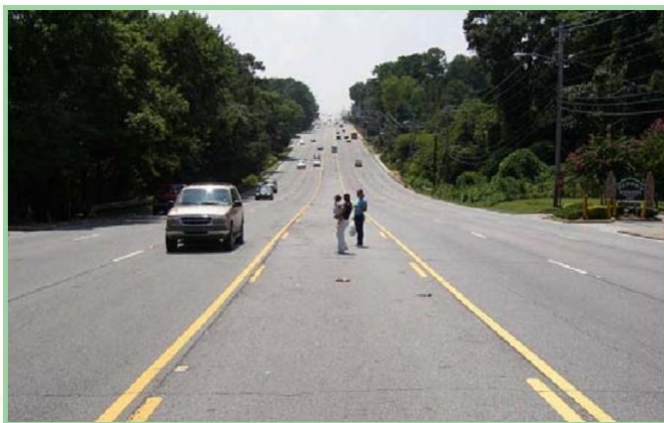
Figure 6 Pedestrian refuge islands break the street crossing into more manageable sections while providing a physical buffer from fast moving traffic. The stop bar is pulled back to help motorists in the inside travel lanes see crosswalk activity. Images courtesy of PBIC.
