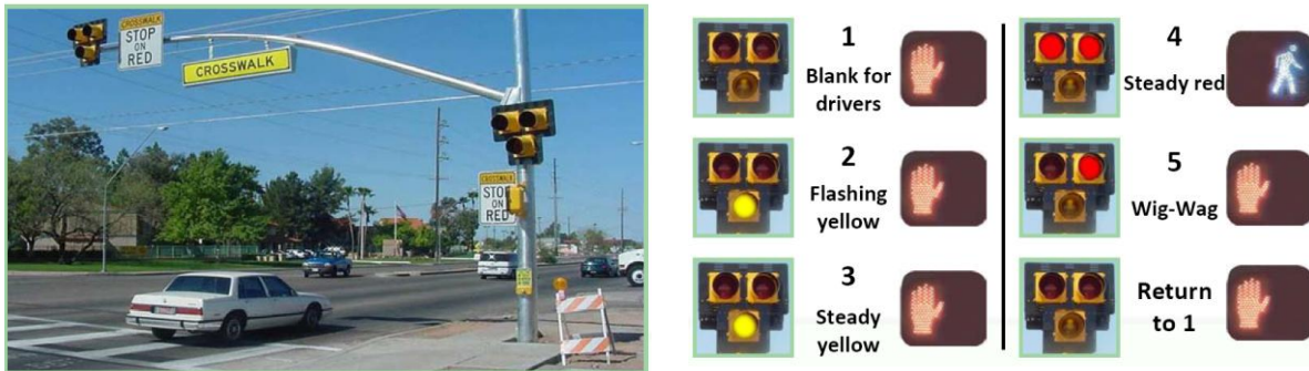
Figure 24 A Pedestrian Hybrid Beacon (or HAWK), included in the MUTCD, helps pedestrians cross busy roads with minimum disruption to vehicular traffic. Images courtesy of PBIC.
