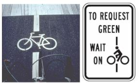
Figure 2.10. Signal activation marking and sign.
