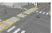
A median refuge area can cut the acceptable gap needed to cross a major street by 50 percent.
