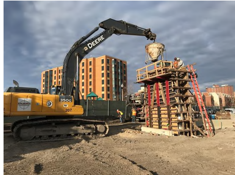
Pier 1 concrete placement. All piers and abutments are installed. Only thrust blocks remain.
