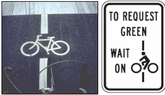
Figure 2.12. Signal activation marking and sign.
